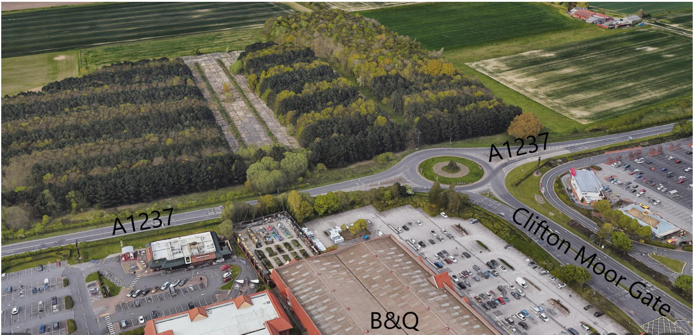
A1237/Clifton Moor Gate Junction (Google Earth)
